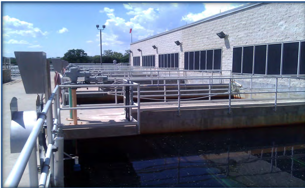
Figure 2: Victoria WTP Filters
