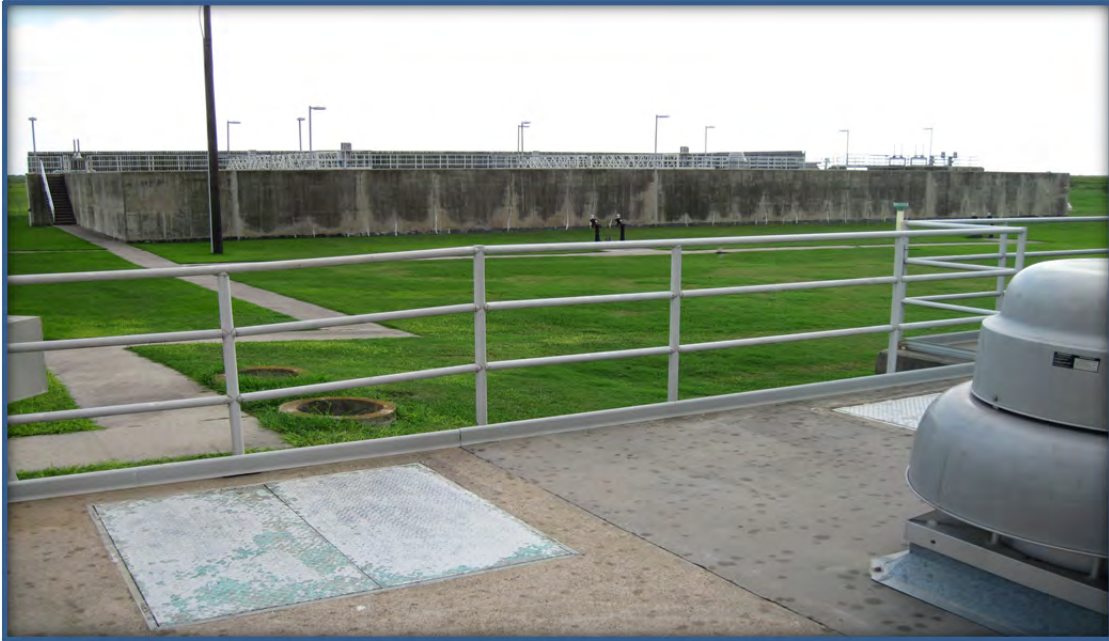
Figure 6: PLWTP Settling Basins
